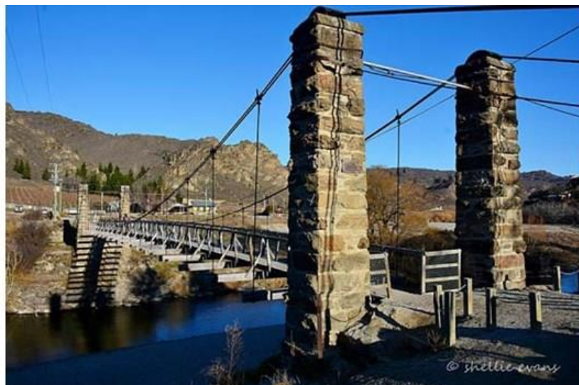
Figure 3. The Manuherikia Suspension Bridge, fondly named Shaky Bridge
