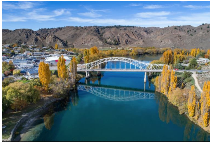
Figure 4. The State highway entrance to Alexandra
