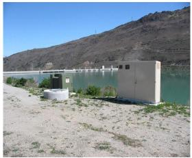
In 2010 the Clyde Water Supply is drawn through schist formations adjacent to Lake Dunstan. The shallow bore is in a screened casing with one submersible pump. Water is pumped to two 1000m<sup>3</sup> concrete reservoirs on the hill above Clyde. Bore water is chlorinated as it enters the reservoir. The shallow bore is considered as an unsecure water source. There is a risk the bore will fail over time due to changes in the water flow path.
